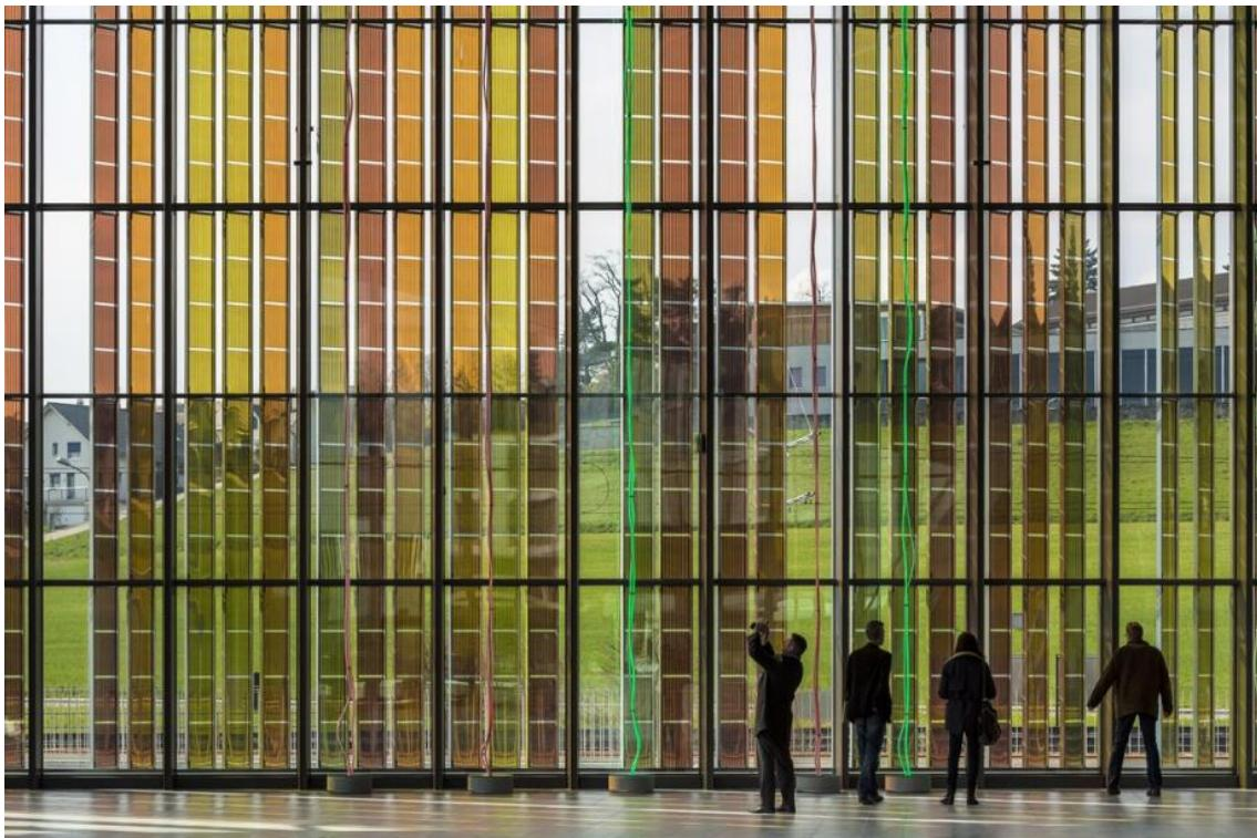
**Sl. 2.5. Stakleni zid prekriven Dye-Sensitized fotonaponskim ćelijama [8]**
