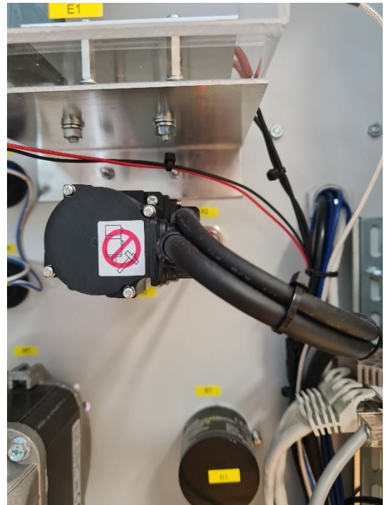
Sl. 2.19 Servomotor HG-KN13J
