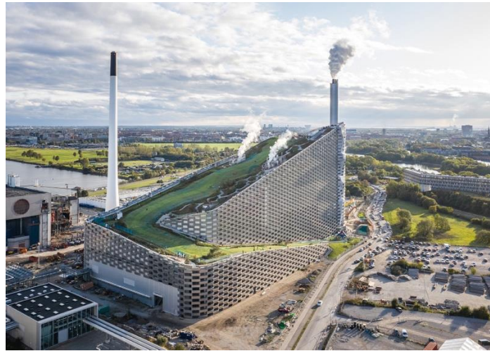
Sl. 4.6 Amager Bakke spalionica otpada u Kopenhagenu [10]
