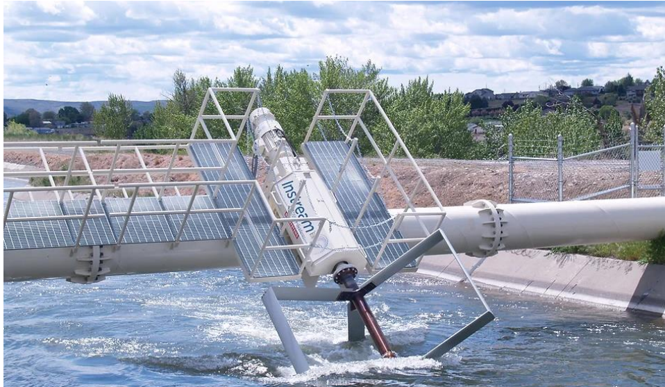
Slika 3.27. Instream Energy Systems H-Darrieusova turbina [36]
