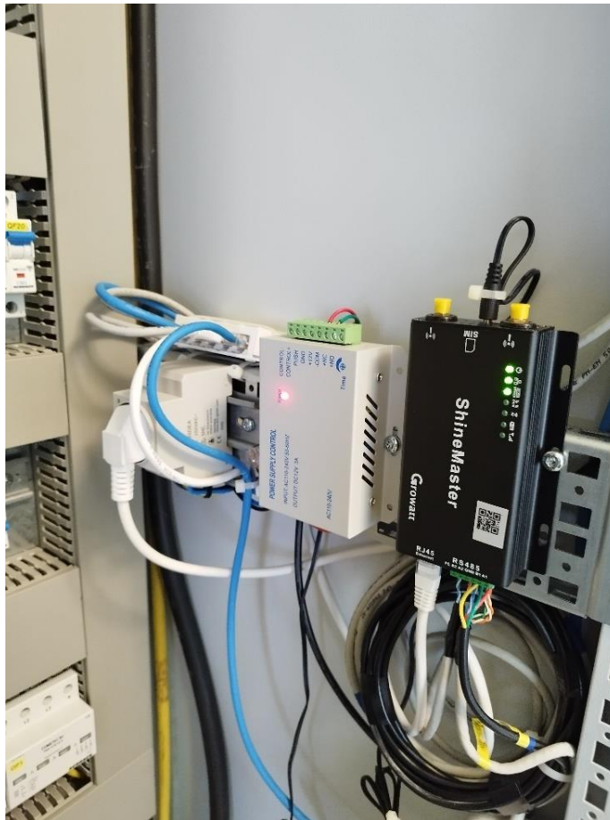
Slika 5.11. Growatt ShineMaster
